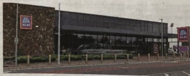
Aldi store on John Joe Sheehy Road, Tralee
